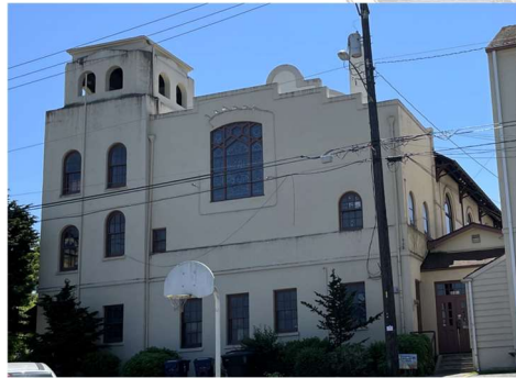
Rear (north) façade, 2023 (Street Alley)
