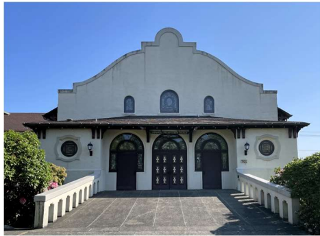
Front (south) façade, 2023 (N J Street)
