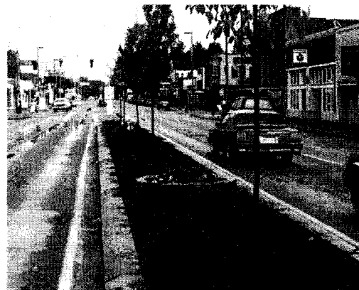
South Tacoma Way Median
