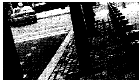
A continuous trench with pavers
