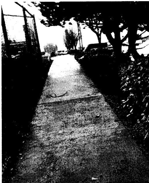
Installation of alternative sidewalk material
