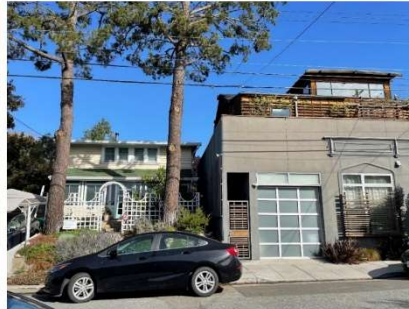
Too close to neighbor, no side yard
