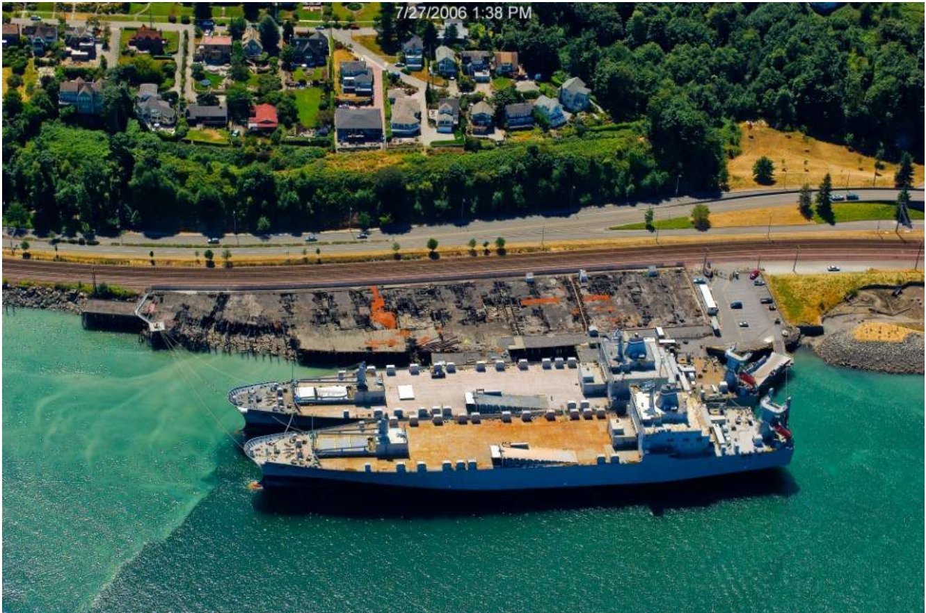
Figure 3-Sperry Ocean Dock (2006) and Tahoma Salt Marsh (r). Most of overwater decking has been removed. 9
