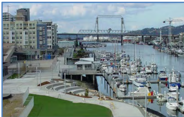
The ABC's of waterfront development: Public esplanade, marinas, and maritime character, linking together restaurants, offices, and retail.
