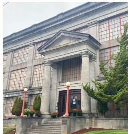
Appendix E Cushman and Adams Substations Feedback Summary Report
