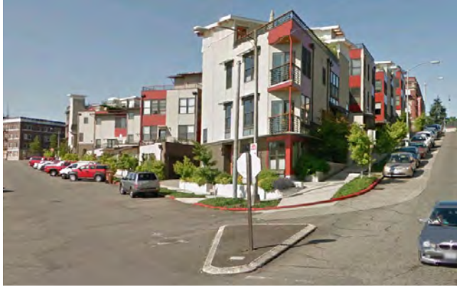
FIG. 2-8 The Triangle Townhomes, a 27-unit condo development in the St. Helens district, is one of the first Built Green projects in downtown Tacoma.
