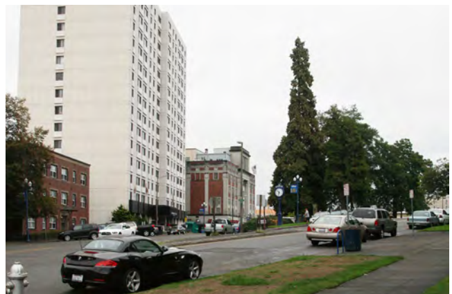
FIG. 2-23 A south-facing view along St. Helens Avenue illustrates the range of mid- and high-rise housing in the St. Helens district.
