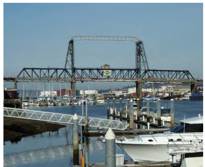
FIG. 2-16 Renovation work on the Murray Morgan Bridge was completed in time to celebrate the structure's 100th anniversary in February of 2013. The bridge serves as an important link between downtown and the Port of Tacoma.
