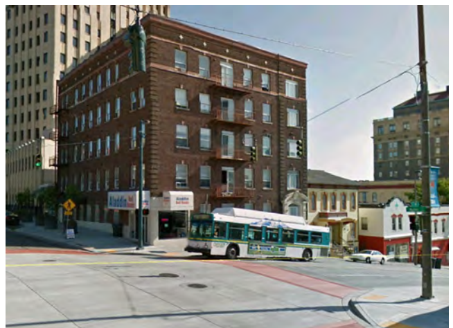
FIG. 6-9 The Rialto Apartments at 311 South 9 th Street.
