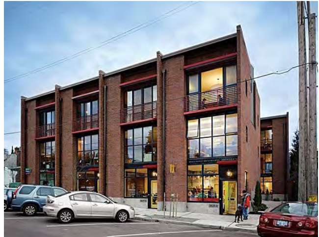
FIG. 3-9 The Columbia City Live-Aboves, an eight-unit project in Seattle, is an example of a live-work unit that provides small business owners with a relatively affordable alternative to traditional mixed use retail space. This adaptable masonry structure was designed to look modern while fitting into the context of a historic neighborhood.
