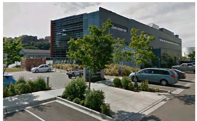
FIG. 2-13 The Center for Urban Waters research facility, located on the east bank of the Foss Waterway, opened after the completion of the Superfund site remediation.
