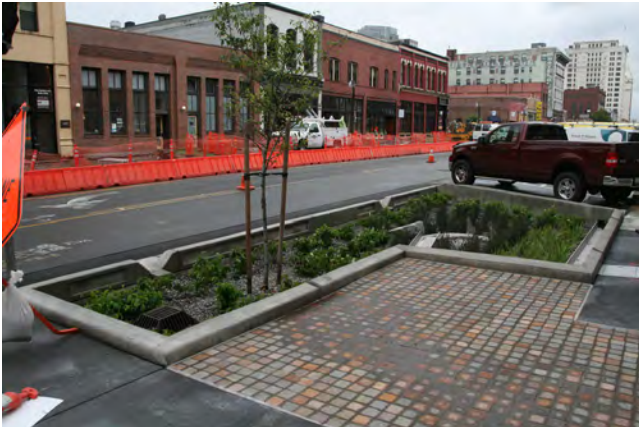
FIG. 8-11 The Pacific Avenue Streetscape project under construction. The project included the addition of fourteen rain gardens to pretreat stormwater before it enters the Thea Foss Waterway.
