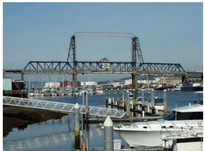
FIG. 8-13 The Murray Morgan Bridge rehabilitation project nearing completion in 2012.
