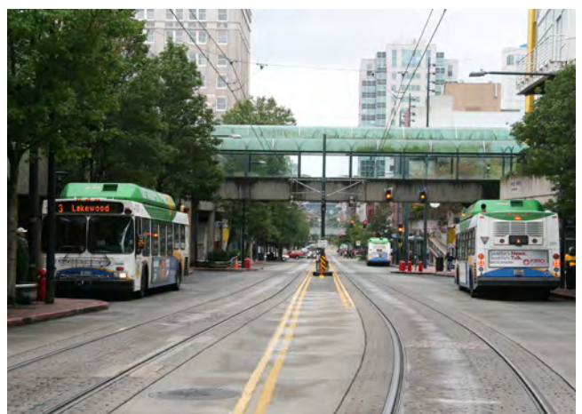
FIG. 2-4 Commerce Street serves as North Downtown's transit hub, providing transit users with an opportunity to make connections between the bus and light rail systems.
