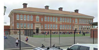
Washington Elementary School in 1949 (above) compared today (below). Source: Northwest Room at The Tacoma Public Library, Richards Studio D44586-3
