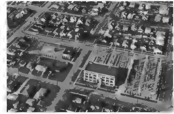
Aerial photo of the Cushman Substation and its various towers in 1963.
