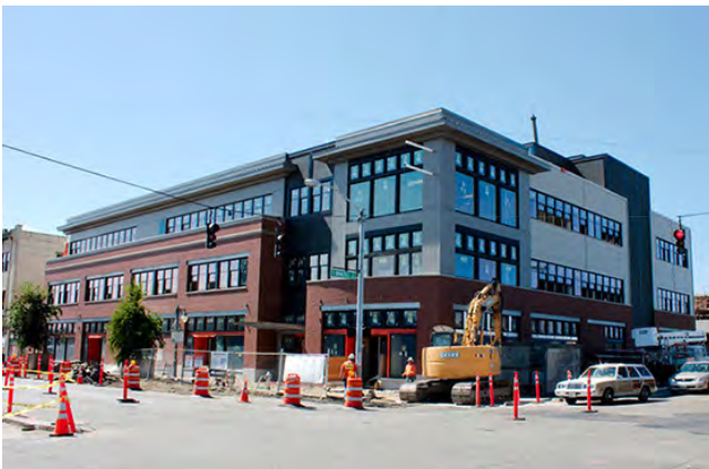
FIG. 2-8 Construction of the new Community Healthcare Clinic on MLK Jr Way.
