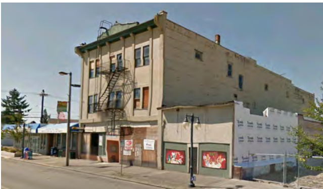
FIG. 7-16 The Tacoma Community Redevelopment Authority (TCRA) recently acquired the Valhalla Hall, a former community social hall in the core of the Hilltop District. TCRA is actively pursuing opportunities for the rehabilitation and adaptive reuse of this historic character building.
