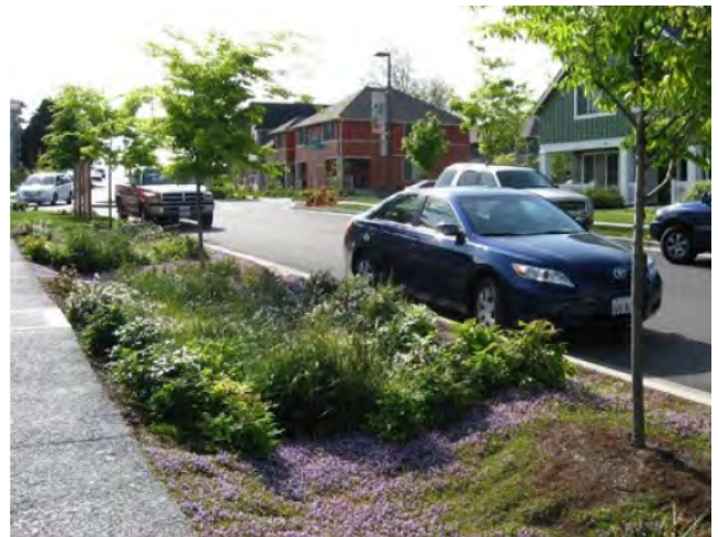
FIG. 4-12 An example of a green street feature, this swale running between the sidewalk and roadway collects and filters stormwater.
