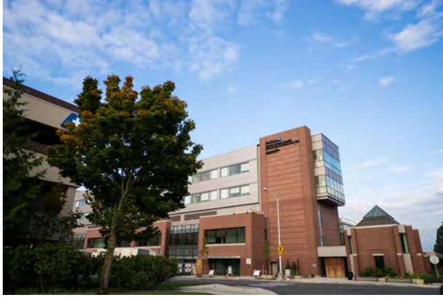
FIG. 2-9 MultiCare's new Milgard Pavilion.
