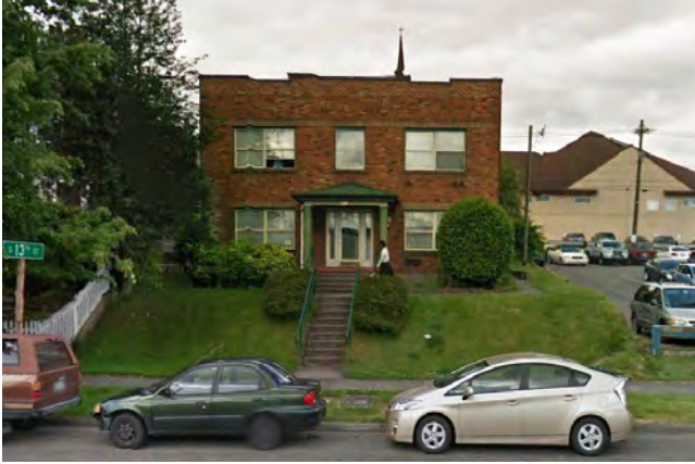
FIG. 3-10 The Campbell Court Apartments on South Yakima Avenue.
