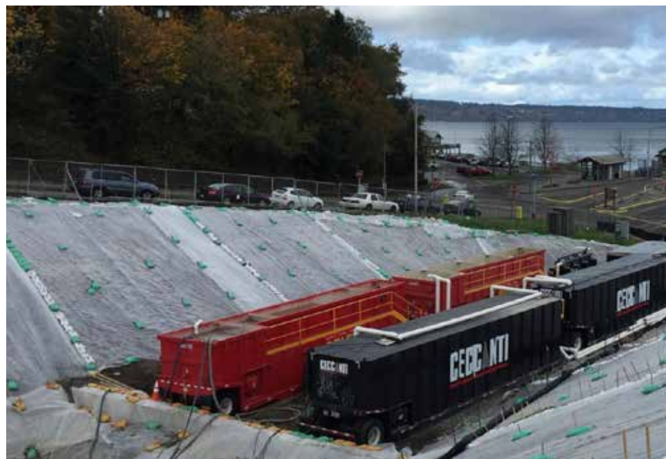
Construction of New Stormwater Facilities at the Triangle
