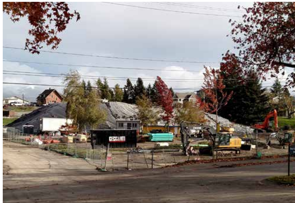
Construction of New Stormwater Facilities at the Triangle
