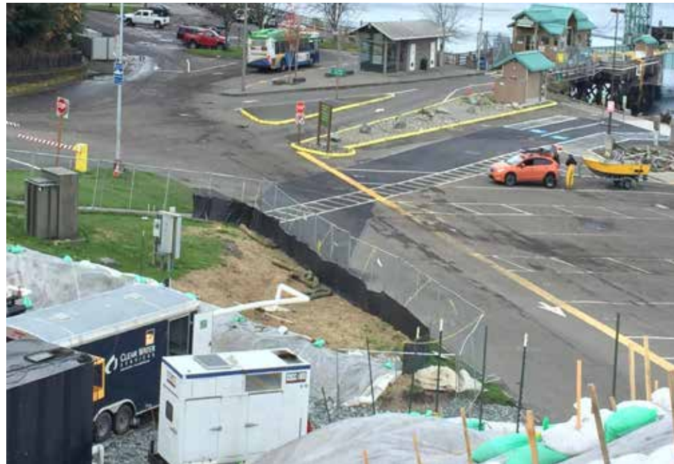
Construction Underway at the Triangle near the Waterfront
