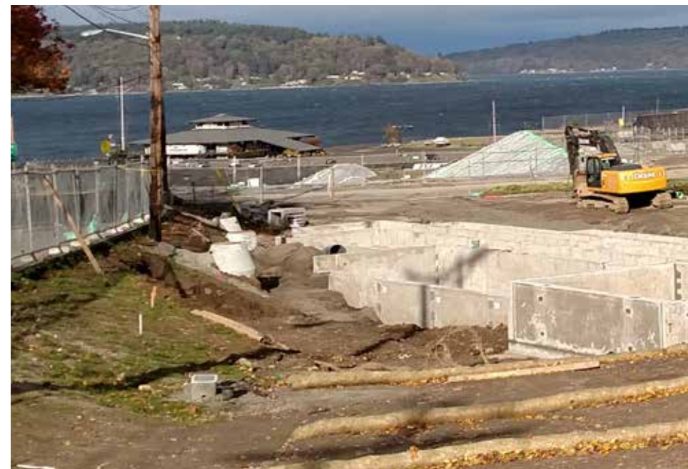
New Stormwater Facilities Being Installed at the Triangle
