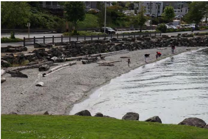
*This soft shoreline along Ruston Way increases public access while also maintaining shore stability through the use of a naturally sloped backshore and anchored logs that stop erosion and allow sediment to travel along the coast naturally.*
