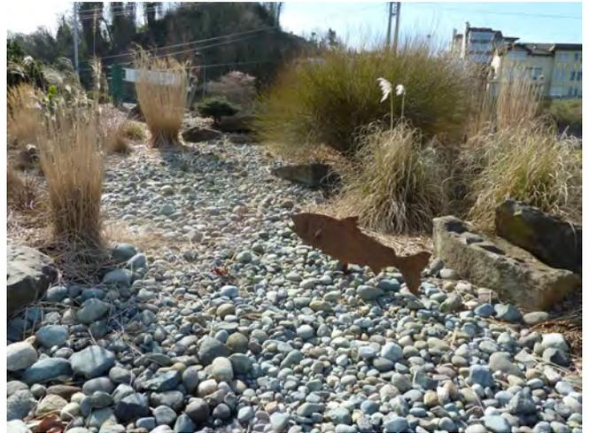
*A stormwater control feature along Ruston Way that directs stormwater runoff from impervious areas and incorporates native plants and artwork.*
