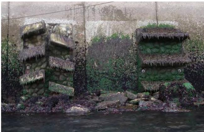
*Microhabitat is created in Puget Sound with habitat panels and troughs attached to the sea wall to provide rough textured surfaces for organisms to attach to despite the hard shoreline.*
