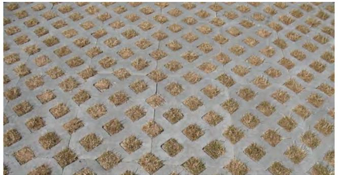
*Permeable pavement allows stormwater runoff to percolate back to the aquifer.*
