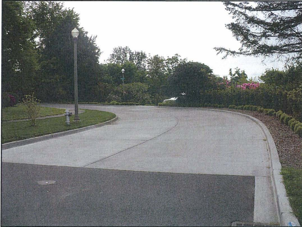
Local Improvement District 7724 Stadium Way looking Northwest to Borough Road
