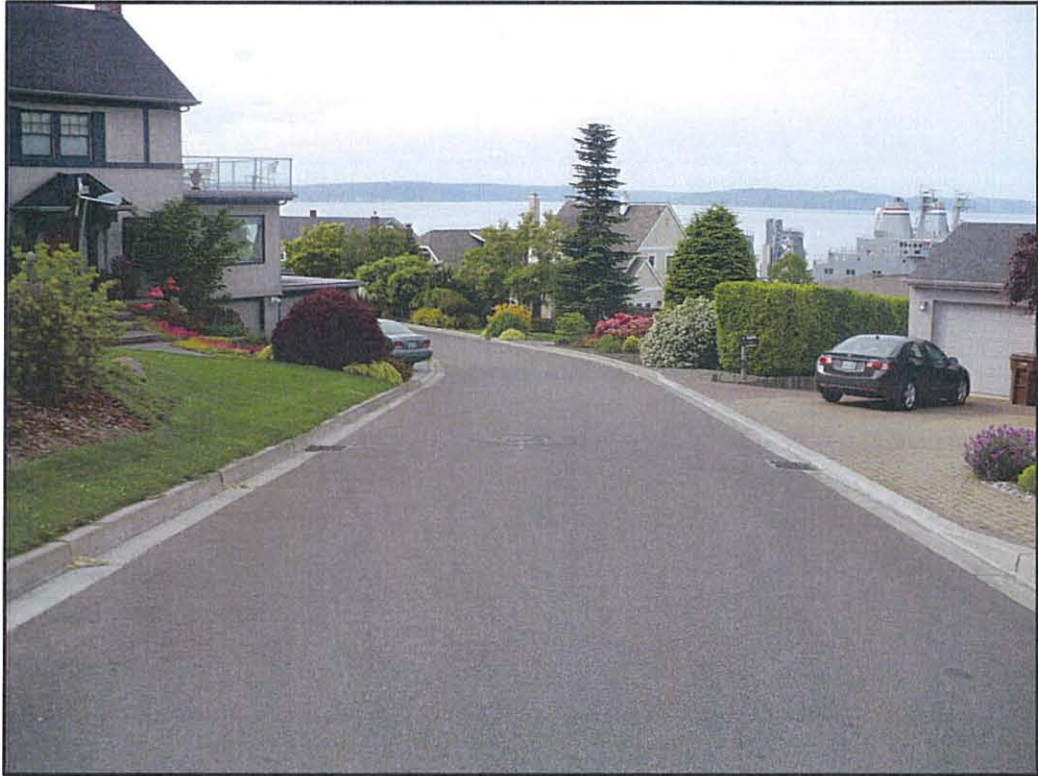
Local Improvement District 7724 Stadium Way looking Northwest from Intersection
