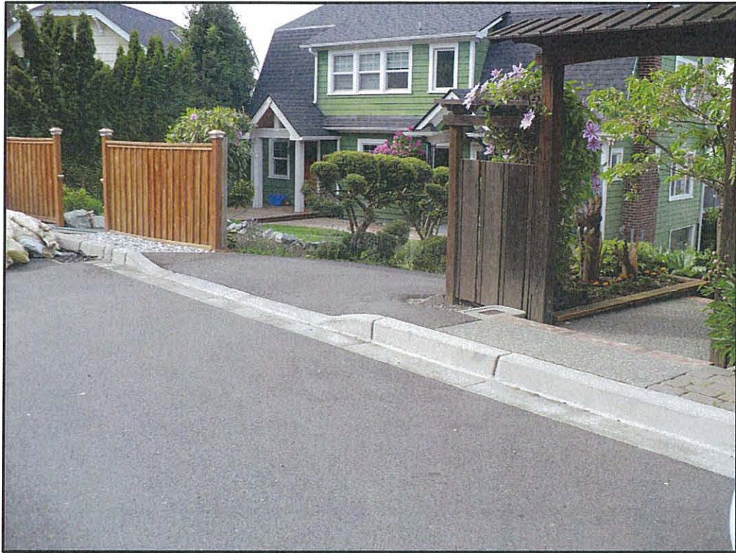
Local Improvement District 7724 Typical View of New Curbing and Gutters
