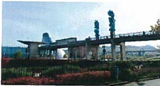
FIG. 9-3 The Bridge of Glass is a key pedestrian connector between the Foss Waterway and Pacific Avenue.
