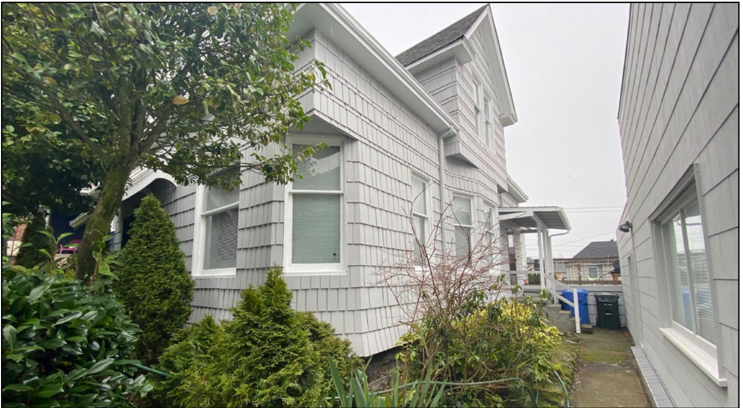
Figure 28 • 205 S Yakima, eastern façade
