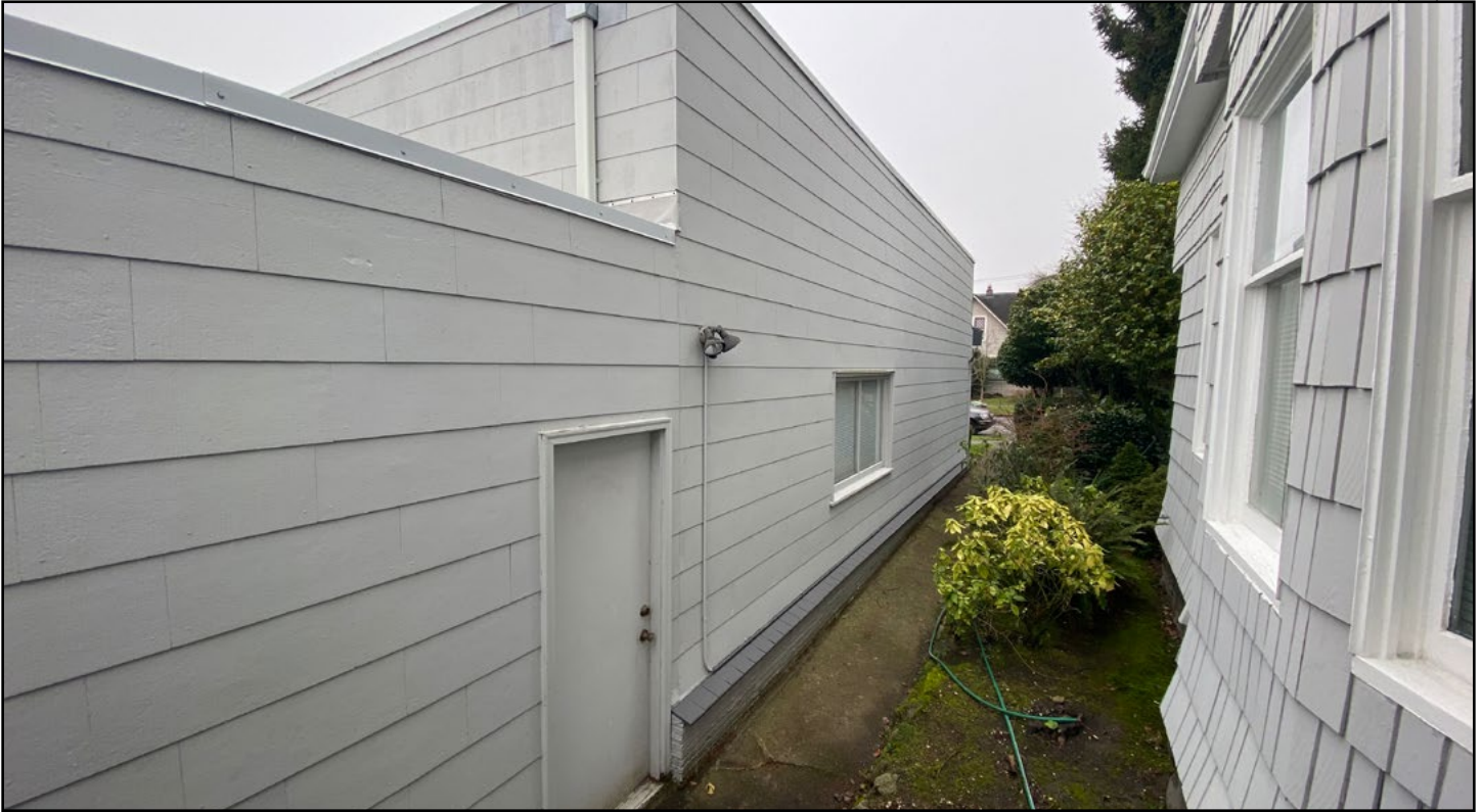
Figure 18 • 201 S Yakima, western façade
