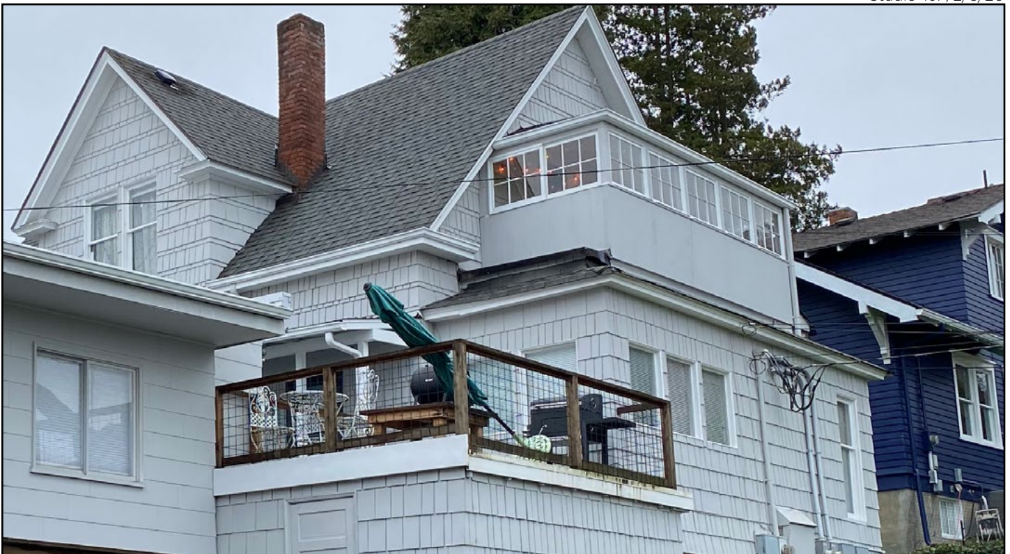
Figure 27 • 205 S Yakima, view from Second Avenue
