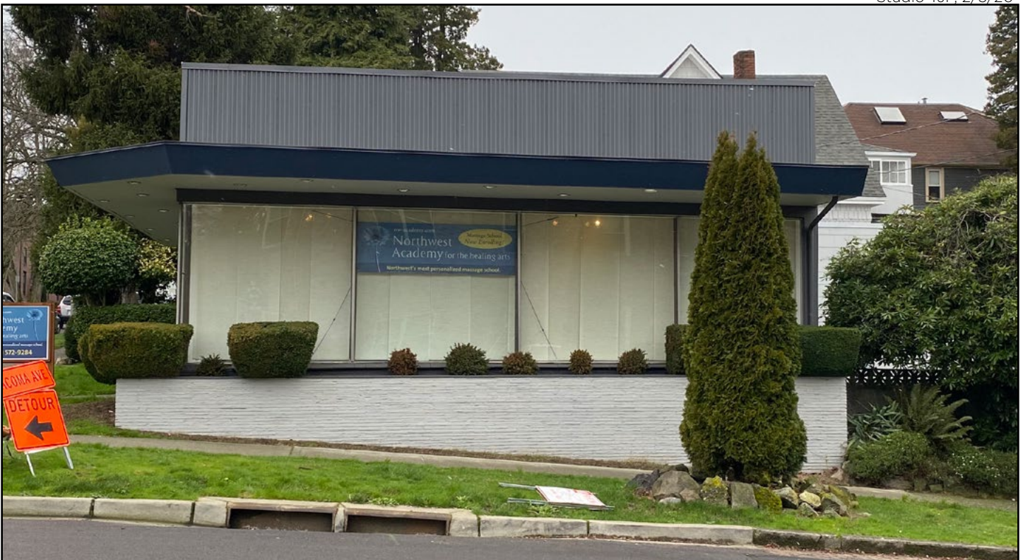
Figure 15 • 201 S Yakima, eastern façade
