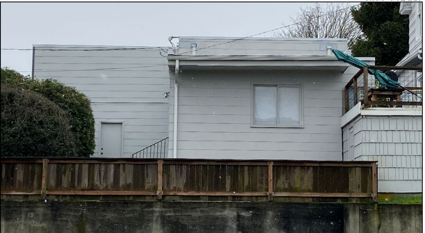
Figure 19 • 201 S Yakima, northern façade
