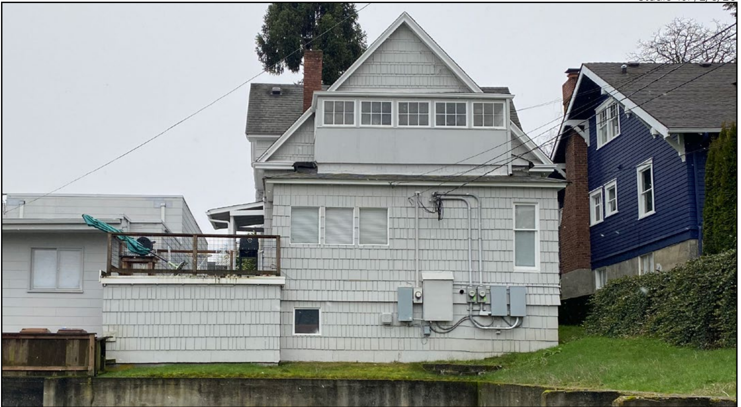
Figure 26 • 205 S Yakima, northern façade
