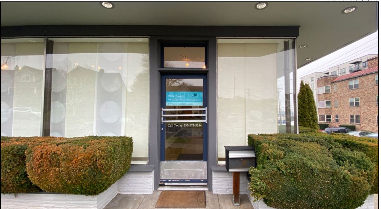
Figure 17 • 201 S Yakima, southern façade detail of entry door
