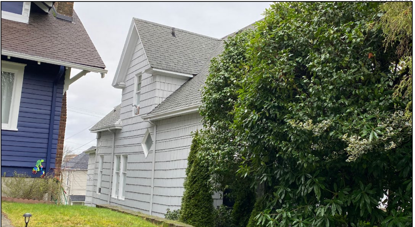
Figure 25 • 205 S Yakima, western façade
