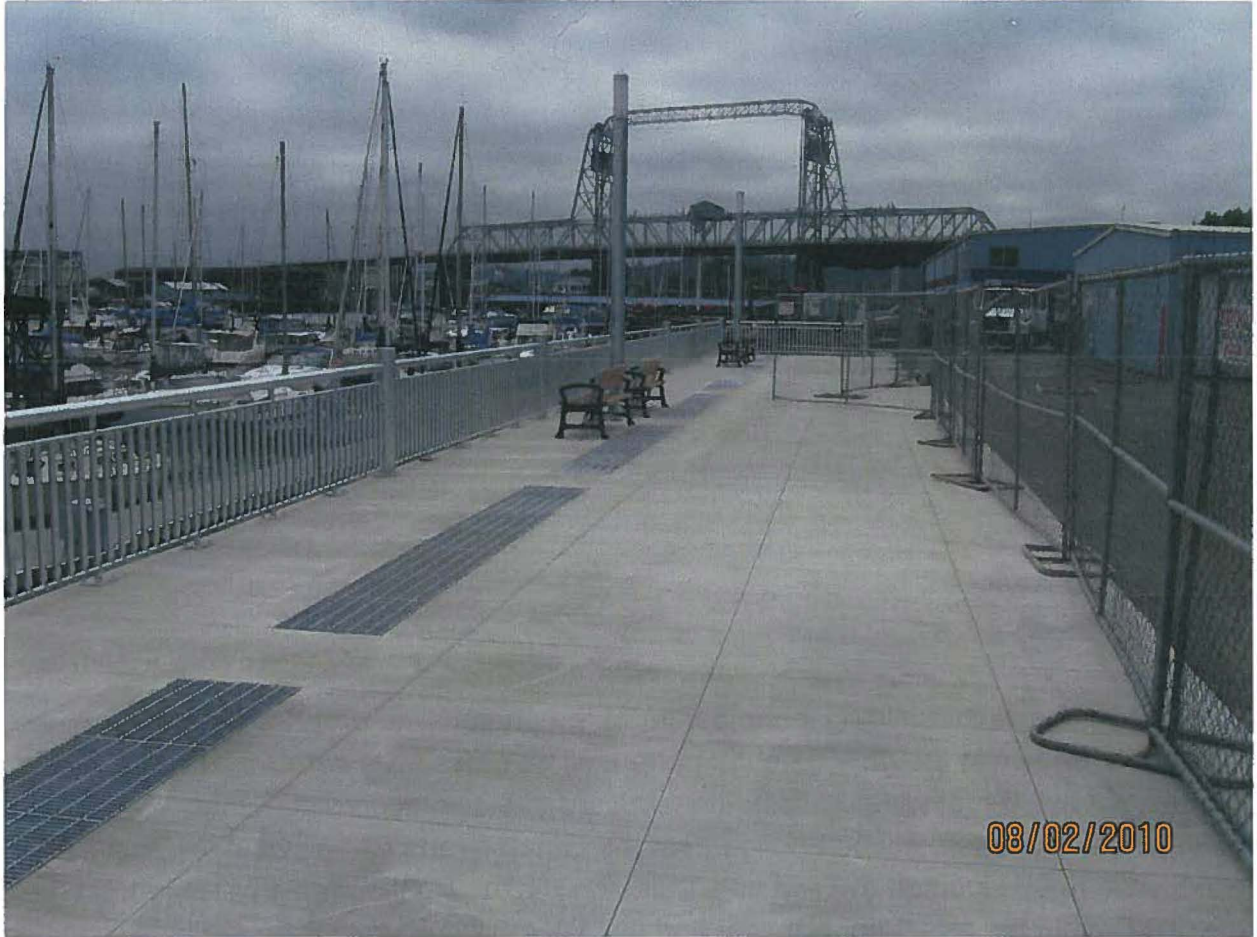
This photo shows the completed Site 11 Phase 1 esplanade project. The Site 11 Phase 2 esplanade will be very similar when completed.
