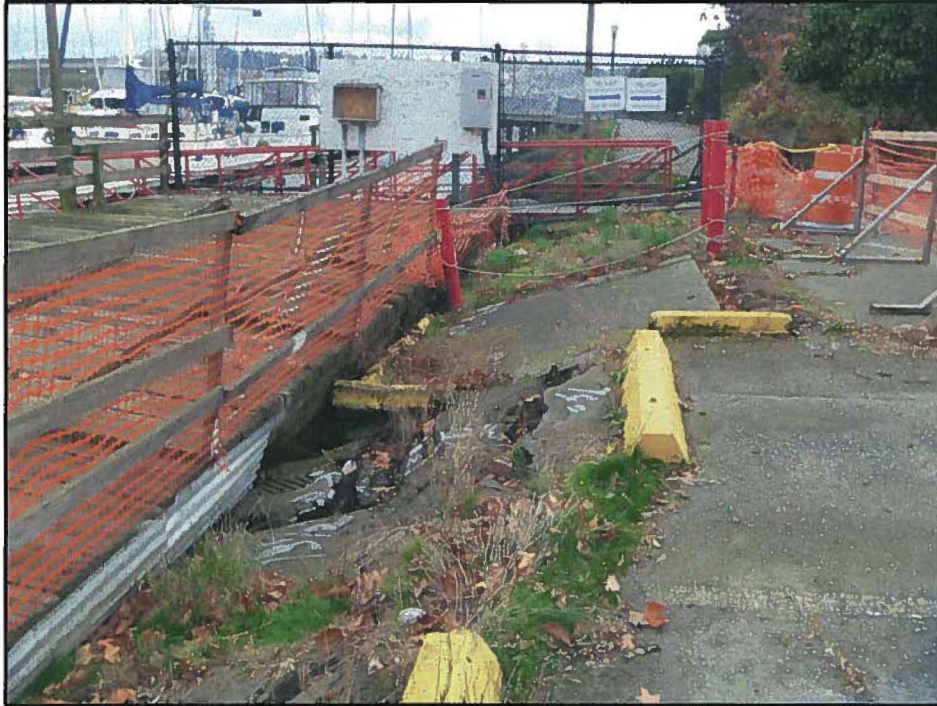
These photos show the failing bulkhead and esplanade structure.
