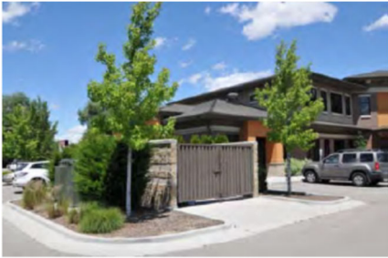
Well-designed service enclosure example.
