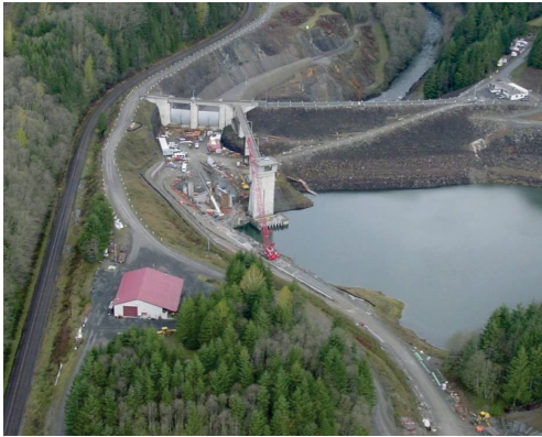
Howard Hanson Dam operated by US Army Corps of Engineers
