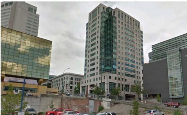
FIG. 4-4 Coordinated Care located its headquarters in the Tacoma Financial Center building in 2013.
