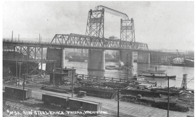
FIG. 5-24 The 11th Street Bridge (later named the Murray Morgan Bridge to honor the local historian) opened on February 15, 1913. The 2,100 foot steel bridge connected the Tideflats to the downtown business district and allowed larger ships to traverse the City waterway.
