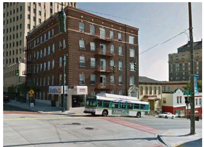
FIG. 6-9 The Rialto Apartments at 311 South 9 th Street.
