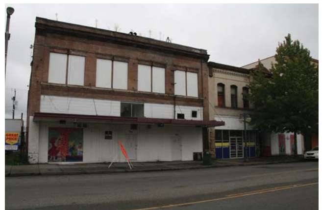
FIG. 4-11 The Kellogg-Sicker and Pochert buildings in the Hilltop neighborhood will be restored to house mixed-use development.
