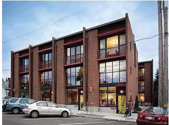
FIG. 3-9 The Columbia City Live-Aboves, an eight-unit project in Seattle, is an example of a live-work unit that provides small business owners with a relatively affordable alternative to traditional mixed use retail space. This adaptable masonry structure was designed to look modern while fitting into the context of a historic neighborhood.
