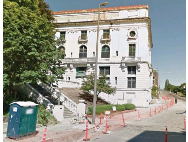
FIG. 4-5 The Elks Lodge building, adjacent to the Spanish Steps, is currently vacant and awaits redevelopment.
