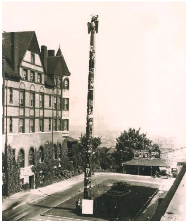
FIG. 5-20 A 1926 photo of the 103-foot Tacoma Totem Pole, one of the City's early landmarks. The totem pole was originally located beside the Tacoma Hotel before its move to Firemen's Park in 1953.
