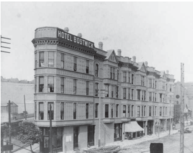
FIG. 5-27 Sited at the prominent intersection of St. Helens and Broadway, the historic Bostwick Building was originally constructed as a hotel.
