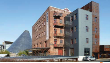
Renovated Albers Mill Lofts building on the Thea Foss Waterway
