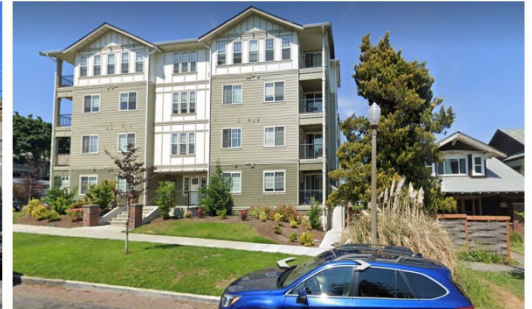
Out of scale with neighboring house
