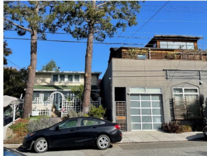
Too close to neighbor, no side yard
