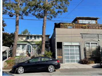
Too close to neighbor, no side yard
