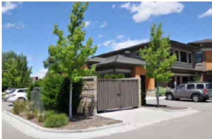
Well-designed service enclosure example.
