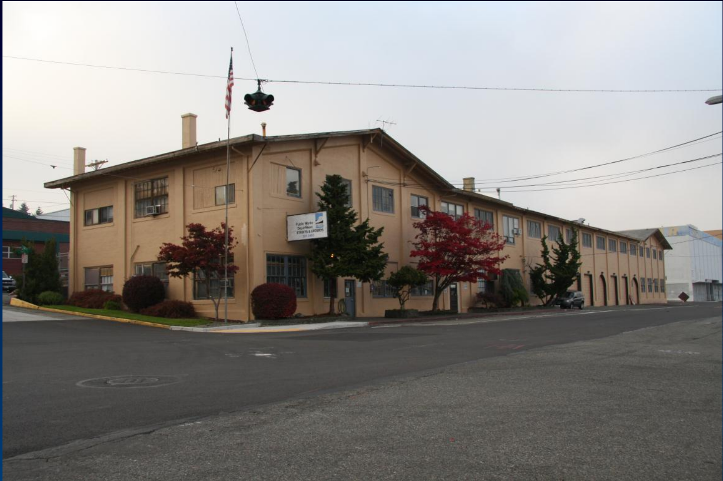
Municipal Barn, Southeast elevation
