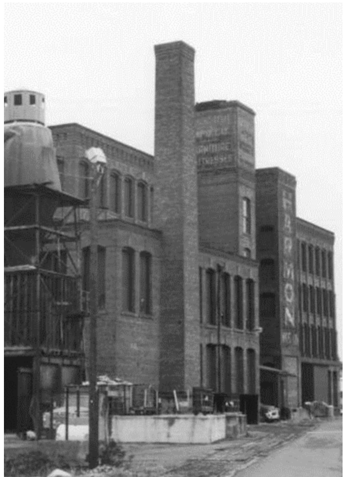
Above: the Willamette Casket Company building, a prominent building in the Nalley Valley, was added to the Tacoma Register of Historic Places in 2023. It will be rehabilitated as maker spaces.
