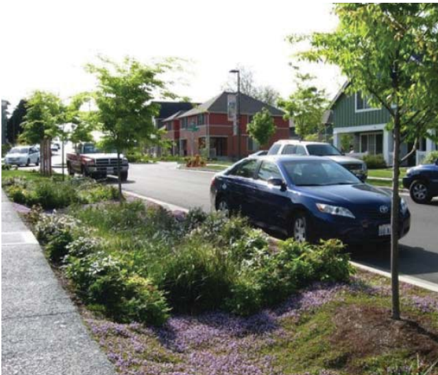
FIG. 8-14 An example of a green street feature, this swale running between the sidewalk and roadway collects and filters stormwater.
