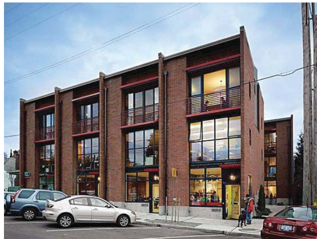
FIG. 4-4 The Columbia City Live-Aboves, an eight-unit project in Seattle, is an example of a live-work unit that provides small business owners with a relatively affordable alternative to traditional mixed use retail space. This adaptable masonry structure was designed to look modern while fitting into the context of a historic neighborhood.
