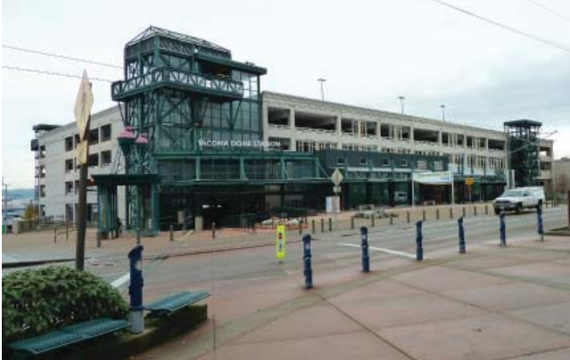
FIG. 9-11 The Tacoma Dome Multimodal Station and parking structure.
