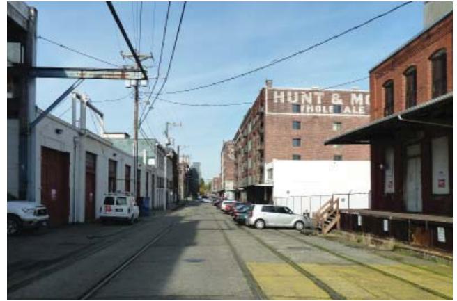
FIG. 2-3 Historic masonry buildings, such as the Hunt Mottet Lofts, contribute to the character of the Brewery District.
