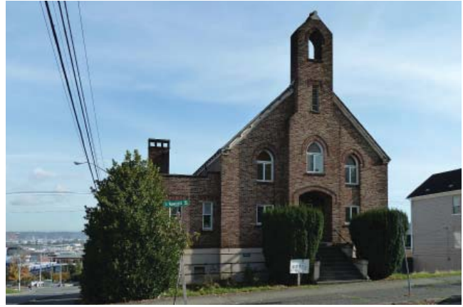
FIG. 2-9 This church on South Fawcett Avenue in the UWT/Museum District has been adapted for use as a dance studio.
