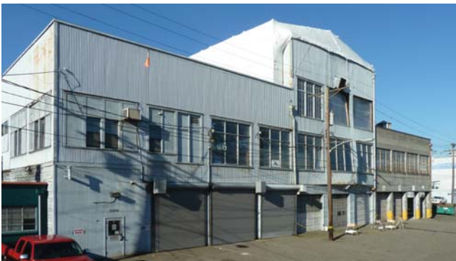
FIG. 11-17 The City Maintenance Building, view from South Holgate Street.
