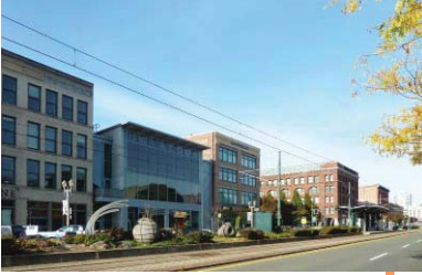
Pacific Avenue, a principal north-south street, in the UWT/Museum District
