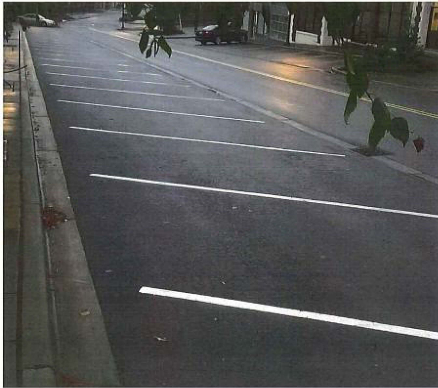
Example of Broadway LID project improvements
