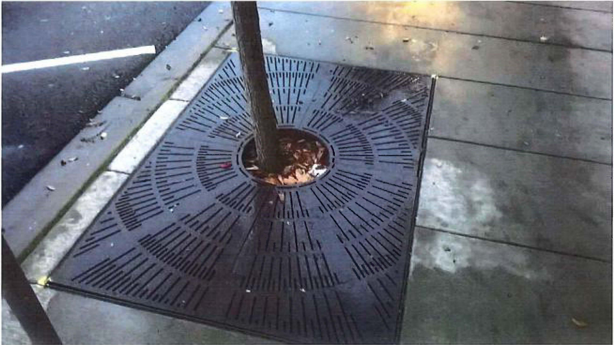
Example of Broadway LID project improvements
