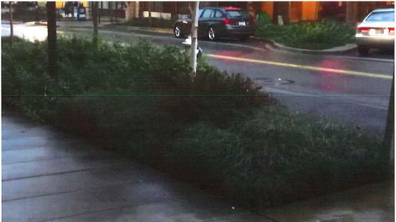
Example of Broadway LID project improvements
