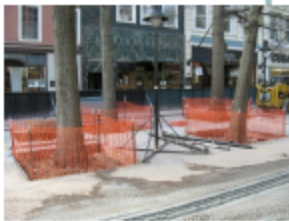
Fencing used around trees to help protect them through construction
