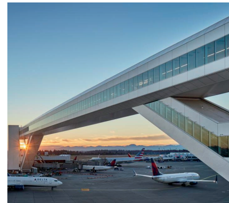
Seattle-Tacoma International Airport (SEA) International Arrivals Facility
