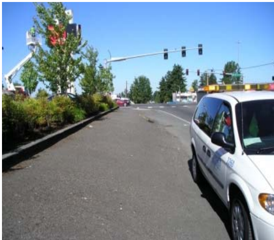
Pre-construction facing west
