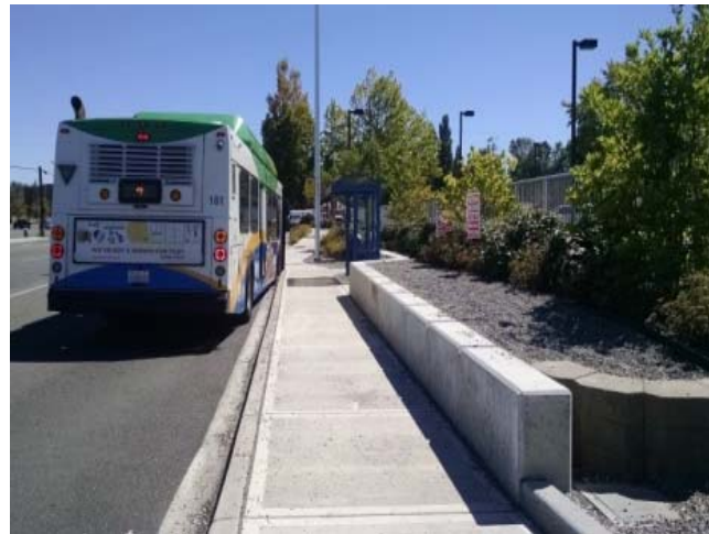
Post-construction facing east
