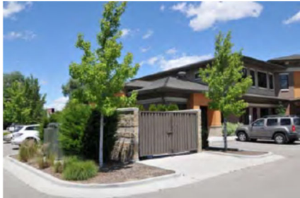
Well-designed service enclosure example.
