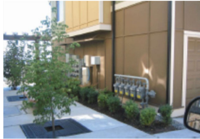
Landscaping helps to minimize the negative visual impacts of utility meters.
