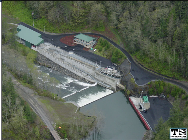
Tacoma - Drinking Water Diversion Dam
