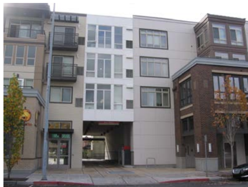
Example of a drive-through within a structure
