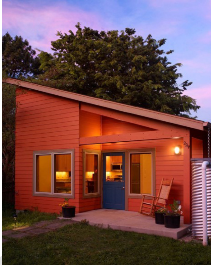
ADU in Portland, OR. Photo Credit: Rainbow Valley Construction.
