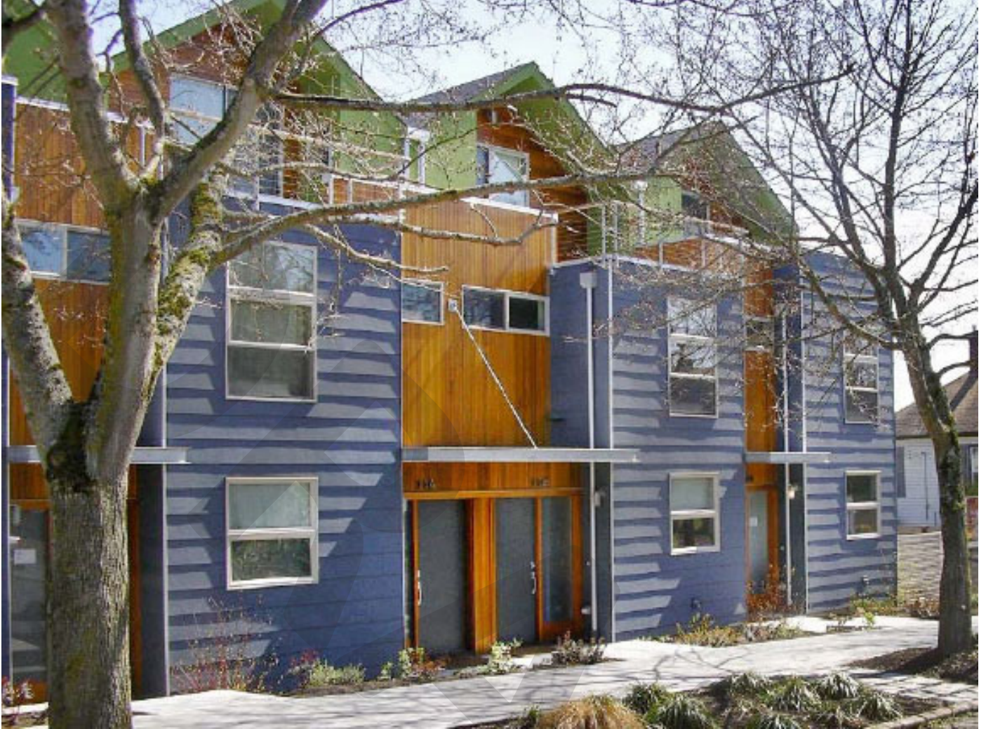
Multi-family development in Seattle, WA. Photo credit: Seattle Department of Construction and Inspections.
