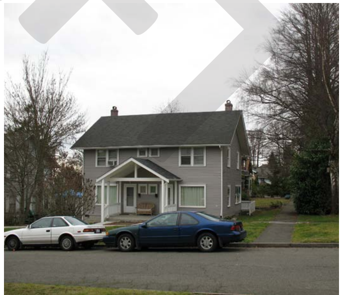
Corner lot duplex in Tacoma, WA. Photo credit: Lauren Flemister
