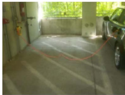
Accessible electric vehicle charging stations may be more cost effectively installed by using an existing end stall or where a clear area is already maintained. Photo source Green Car Reports
