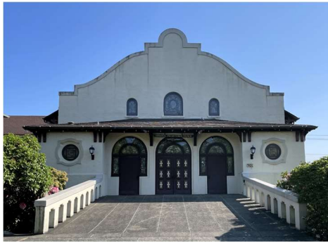
Front (south) façade, 2023 (N J Street)
