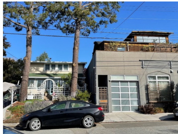
Too close to neighbor, no side yard
