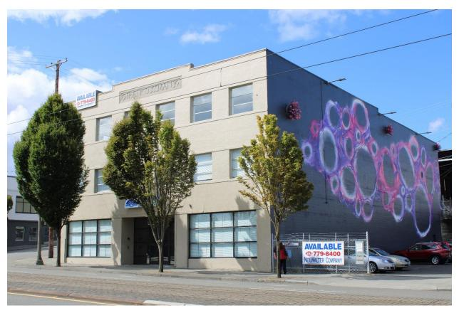
Constructed in 1930 for the Frank Sussman Steel Supply firm, the Sussman block is 120 x 65 and is made from poured in place concrete protecting a steel frame. The building is three stories tall. Sussman was a dealer is government surplus items. After World War Two, the building was the location of several moving and storage companies. The building currently houses a social services provider.
