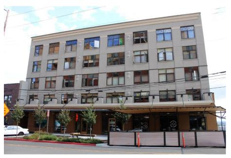
This newly completed Hunt Mottet warehouse was constructed in 1906 with three stories and plans for additional floors above. In 2020, more than a century later, the upper four floors were completed using Cross Laminated Timber (CLT)
