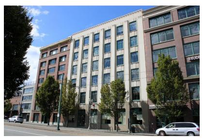
Built concurrently with the Morris Miller Building, the Tacoma Grocery has been inexplicably altered. The alterations were necessary after an unfortunate incident with a failed fire suppression system caused the six-story façade of the structure to collapse in the 1940s. The historic brick façade was replaced with concrete in an
